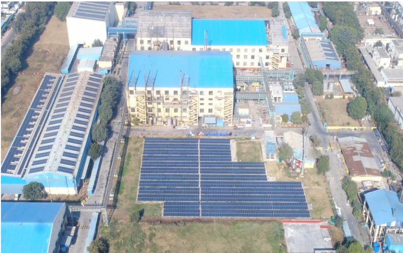
Solar Panel installation at Bawal Plant
